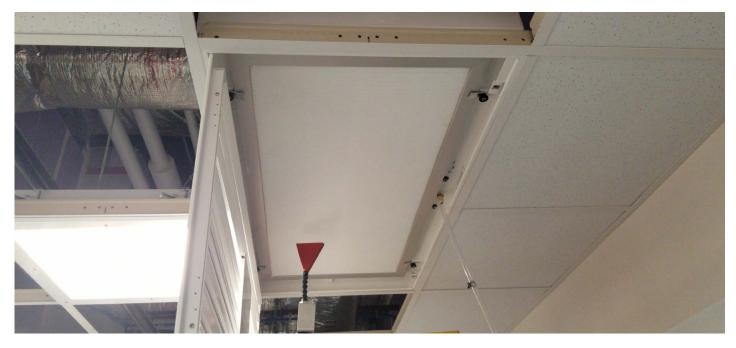
**Step 5:** Disconnect the test equipment, reinstall the plug in the aerosol injection port and reinstall the diffuser face. If the safety cables were disconnected when removing the face, they must be reattached. Make sure all fasteners are firmly latched.
